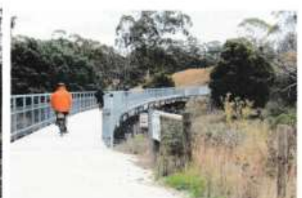
Across one of the bridges
